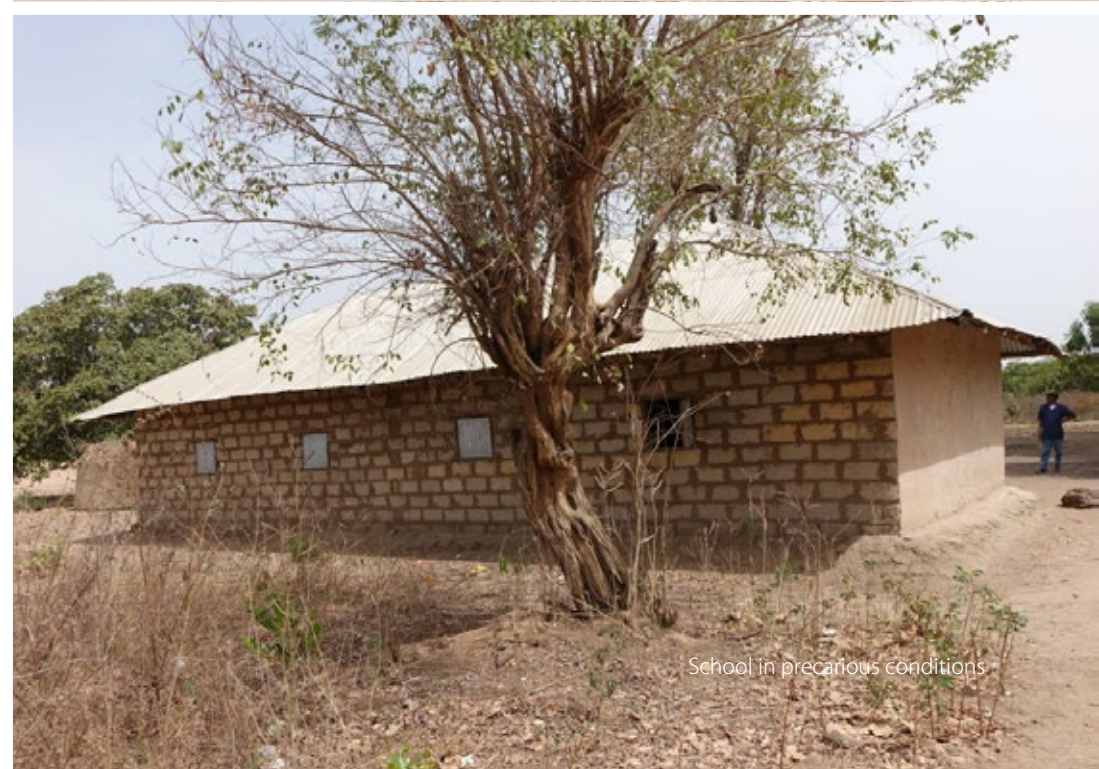
Extension of a school with temporary classes
